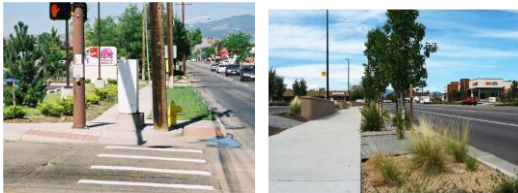
Buried power lines
